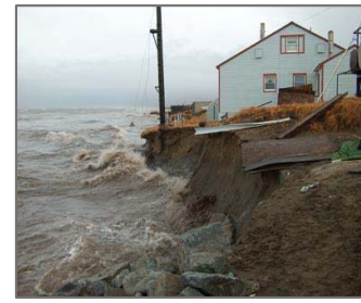
Shishmaref, AK. Source: Shishmaref Erosion and Relocation Commission
