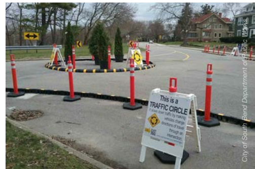
Temporary traffic circle installation, prior to painting
