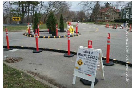
Temporary traffic circle installation, prior to painting
